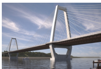
Ohio River Bridges US
